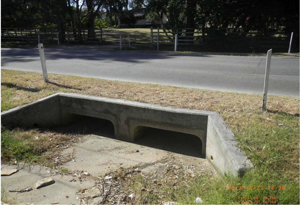
Inlet of Formosa Road culverts (Left culverts)
