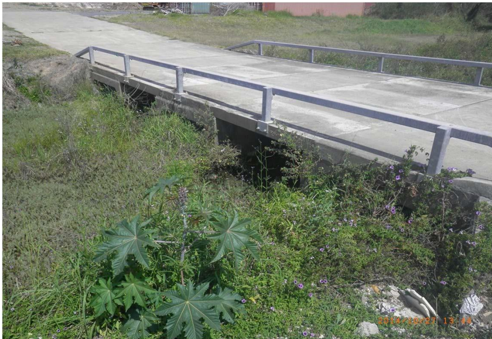
Outlet of culverts at 98 Ingleston Road
