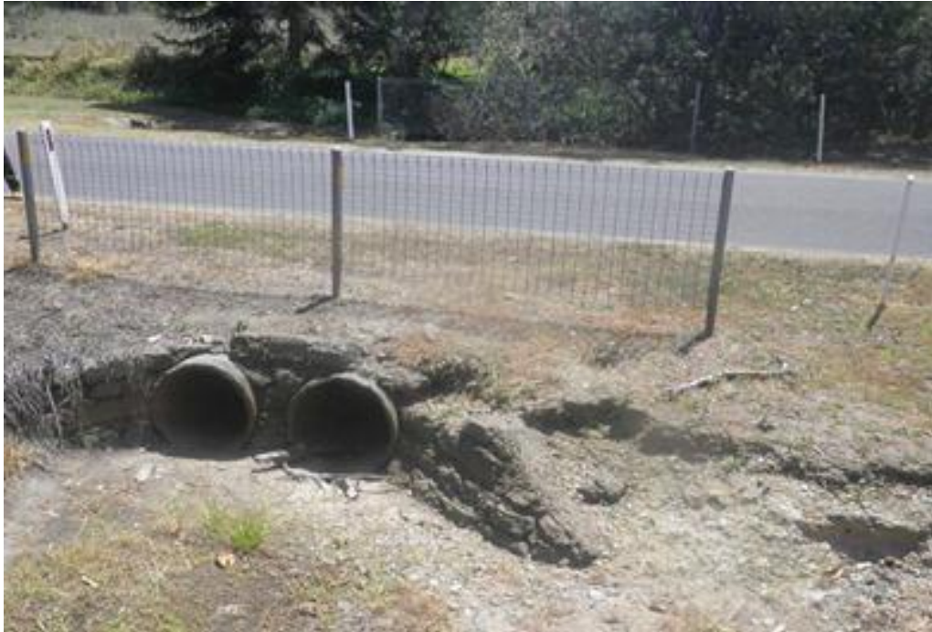
Inlet of Boston Road culverts (London Branch)
