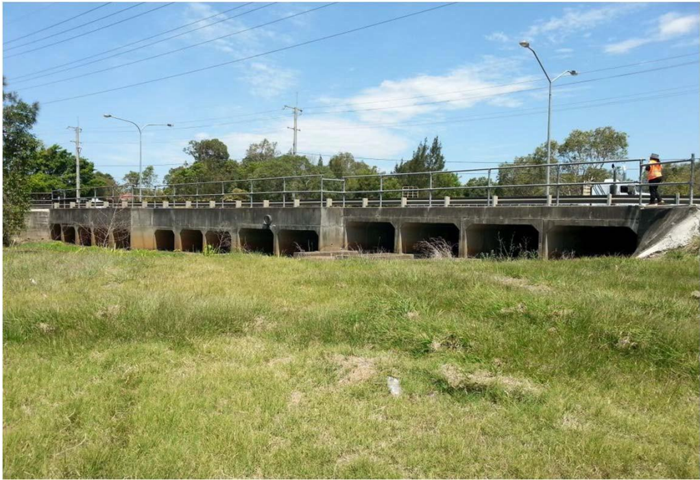
Outlet of Manly Road culverts (Tingalpa Channel)
