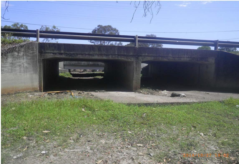
Outlet of Wynnum Road culverts (West Branch)
