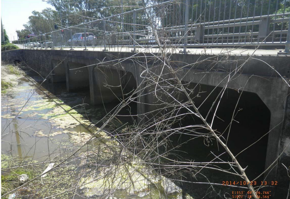
Inlet of culverts at Manly Road
