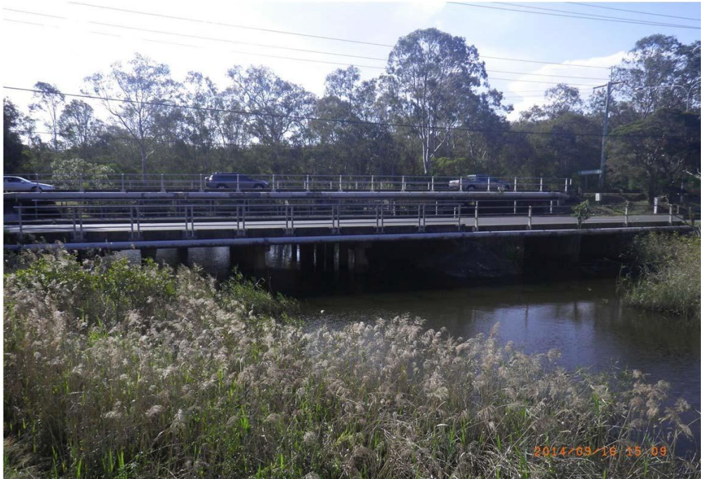
Inlet of Wynnum Road bridge/culverts
