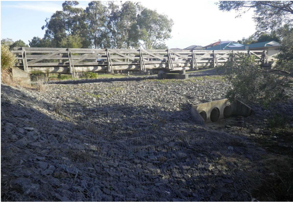
Outlet of culverts and spillway from detention basin
