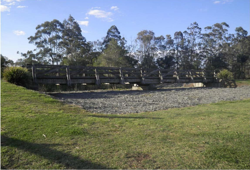
Spillway at detention basin (culvert inlet not visible in photo)
