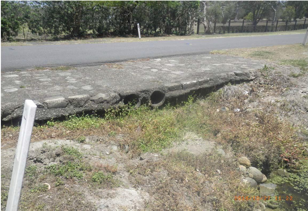
Outlet of Boston Road culverts (East Branch)
