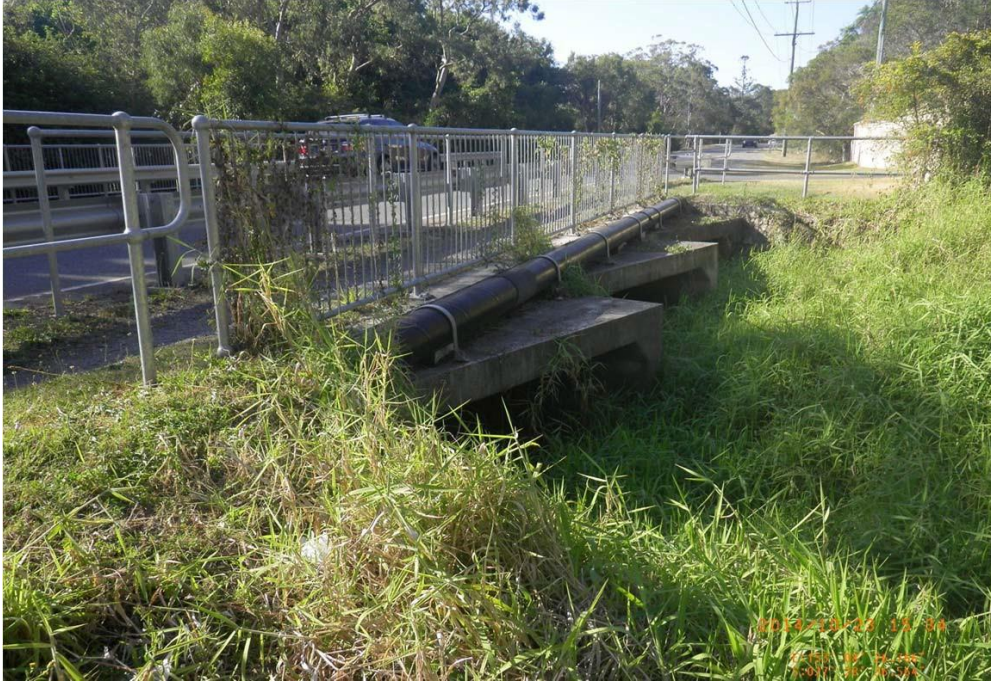
Inlet of Stanbrough Road culverts (East Branch)
