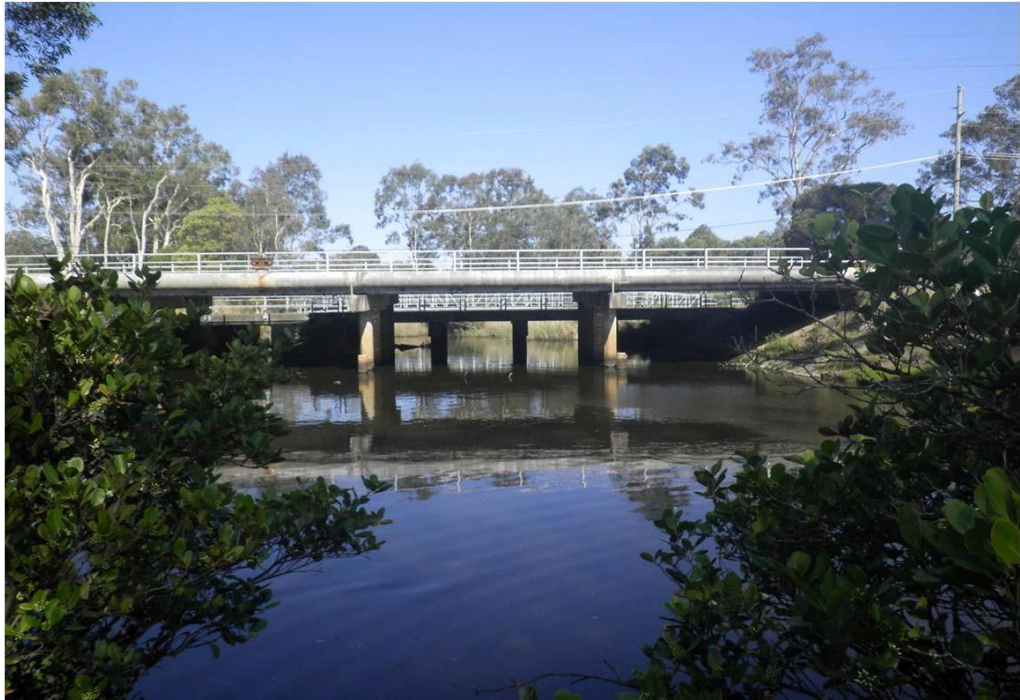
Outlet of Wynnum Road bridge/culverts
