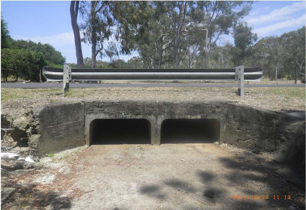
Outlet of Boston Road culverts (East Branch)
