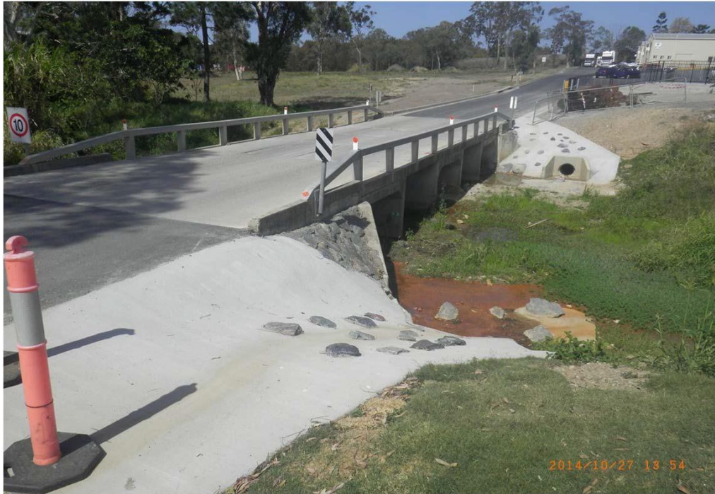
Inlet of culverts at 84 Ingleston Road
