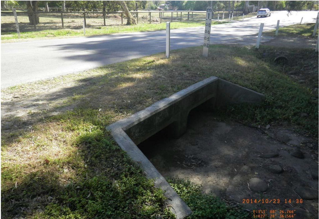
Outlet of Formosa Road culverts (Left culverts)
