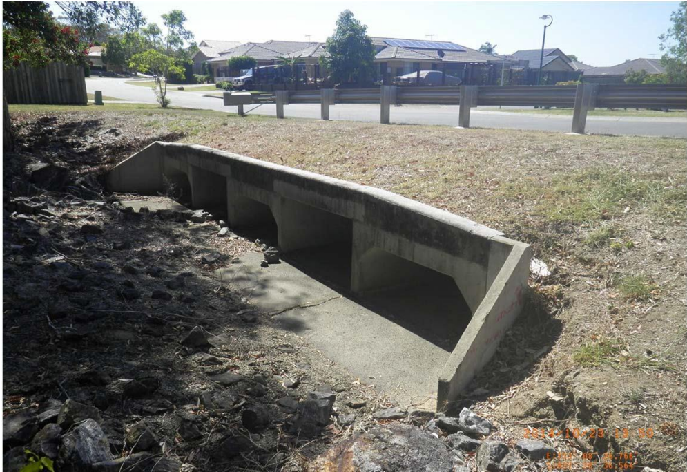
Inlet of Matthews Way culvert (1st Crossing)
