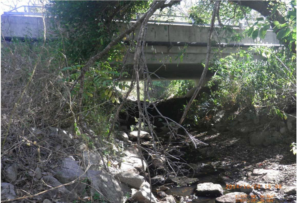
Outlet of Grassdale Road Bridge
