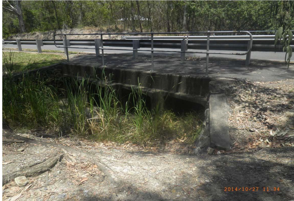
Outlet of London Road culverts (London Branch)
