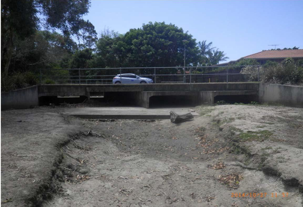
Inlet of Matthews Way culvert (2nd Crossing)
