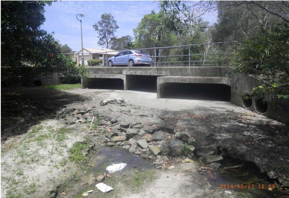
Outlet of Matthews Way culvert (2nd crossing)
