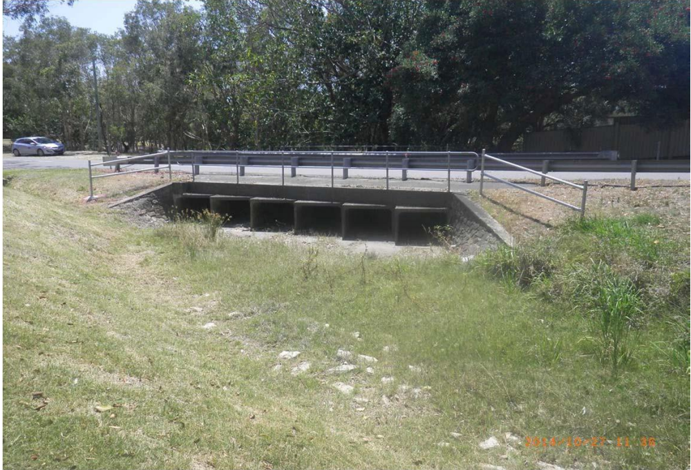
Inlet of London Road culverts (Tingalpa Channel)
