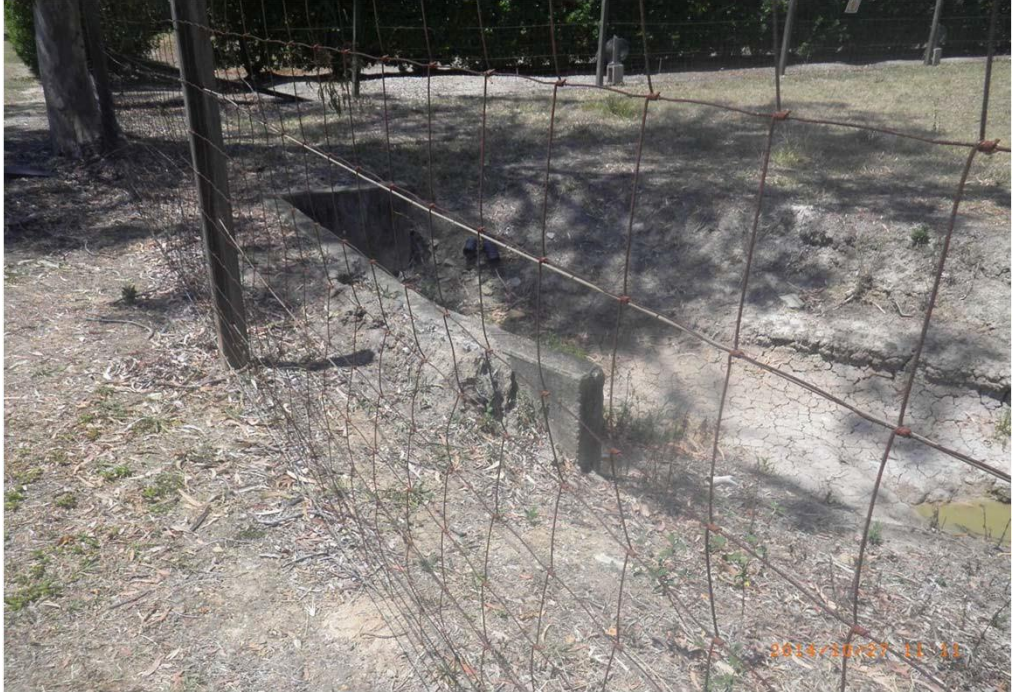
Inlet of Boston Road culverts (East Branch)
