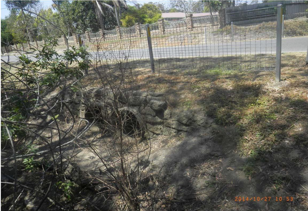
Outlet of Boston Road culverts (London Branch)
