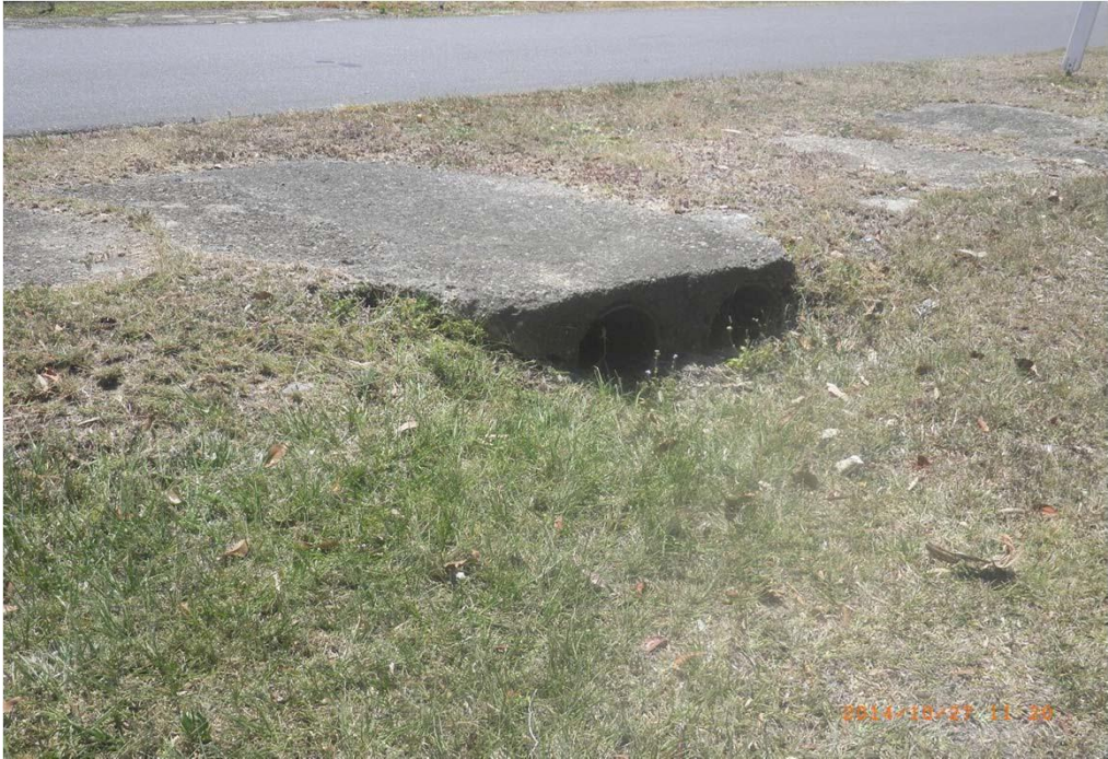
Inlet of Boston Road culverts (East Branch)
