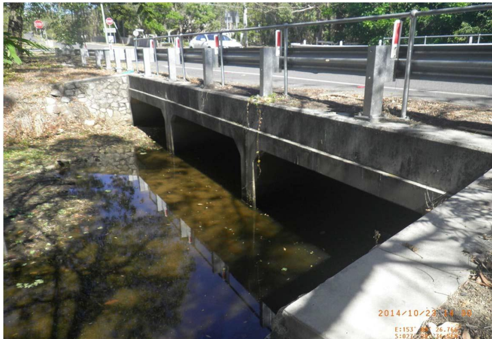
Outlet of Formosa Road culverts (East Branch)
