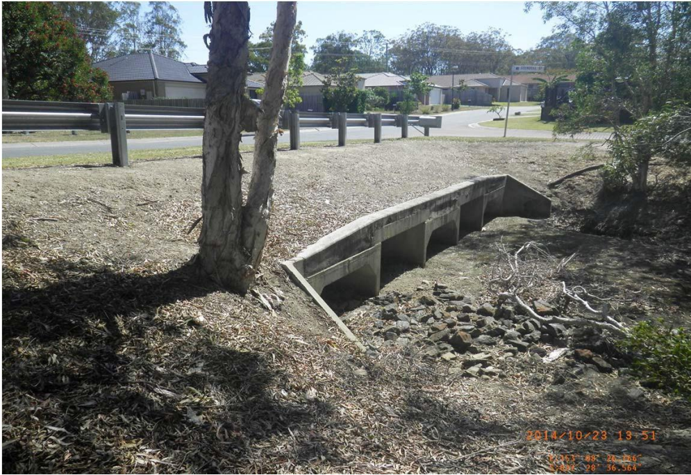
Outlet of Matthews Way culvert (1st Crossing)
