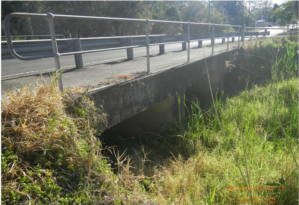
Outlet of Grassdale Road culverts (East Branch)
