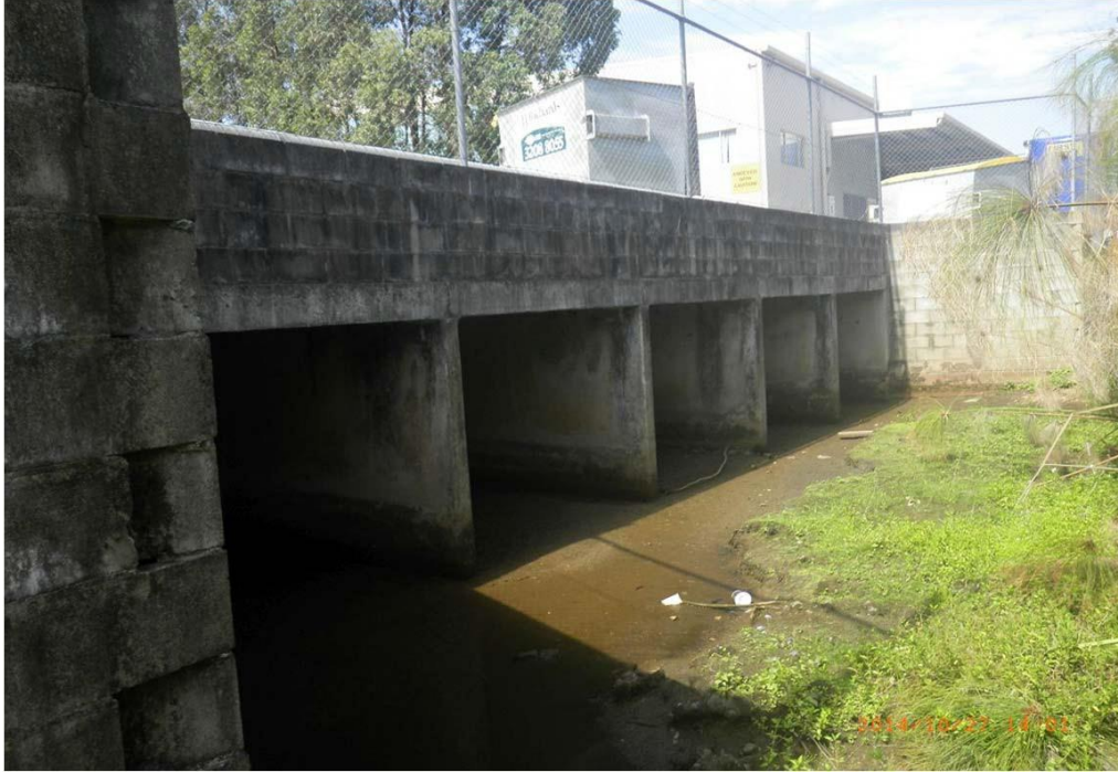
Inlet of culverts at 56 Ingleston Road
