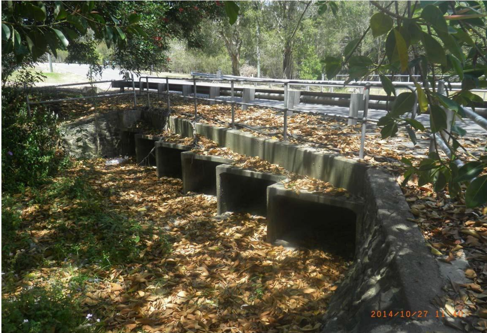
Outlet of London Road culverts (Tingalpa Channel)
