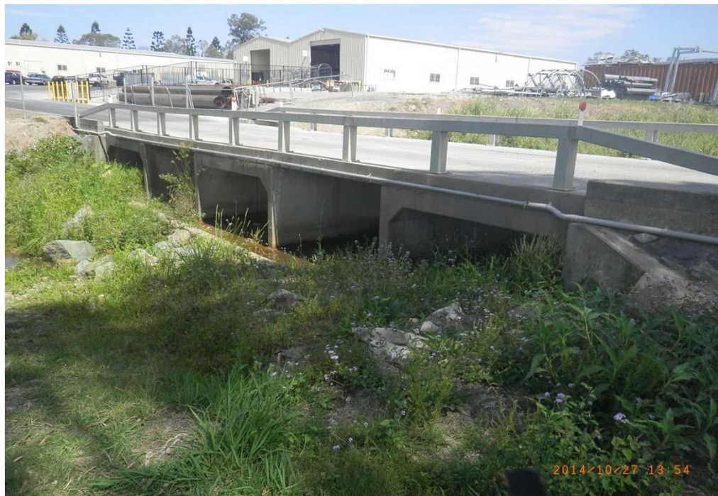
Outlet of culverts at 84 Ingleston Road
