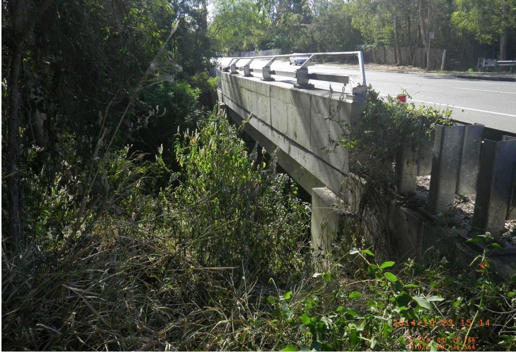
Inlet of Grassdale Road Bridge
