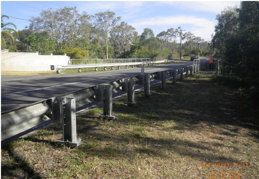
Outlet of Stanbrough Road culverts (East Branch)
