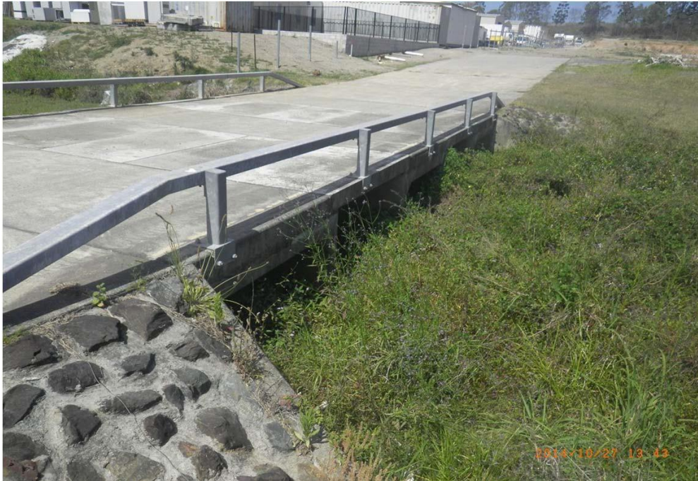
Inlet of culverts at 98 Ingleston Road
