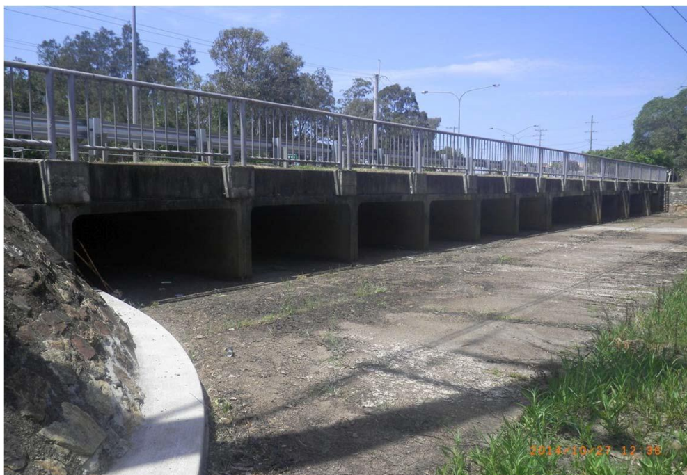
Inlet of Manly Road culverts (Tingalpa Channel)
