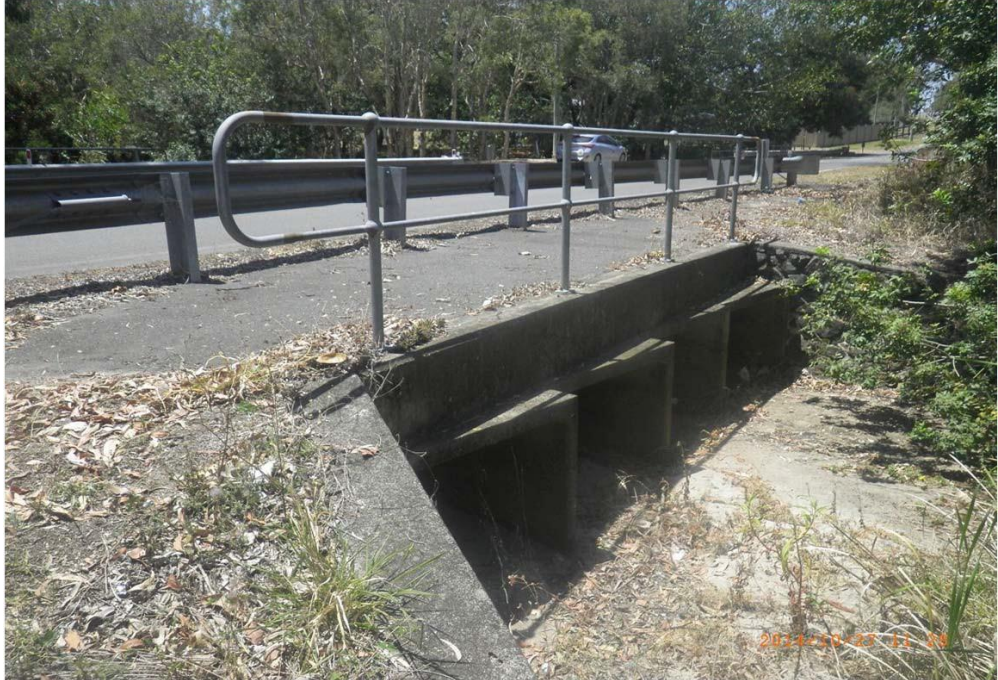
Inlet of London Road culverts (London Branch)
