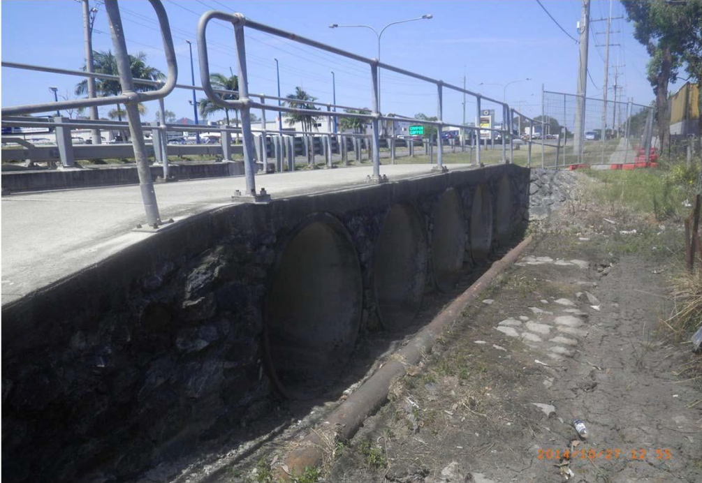
Inlet of Wynnum Road culverts (West Branch)
