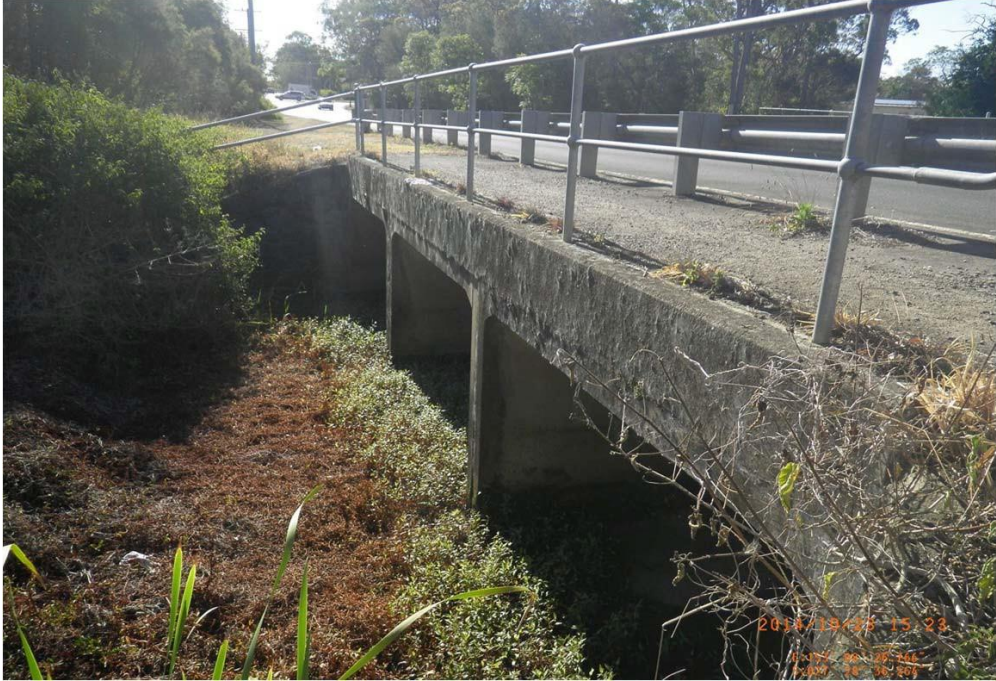
Inlet of Grassdale Road culverts (East Branch)
